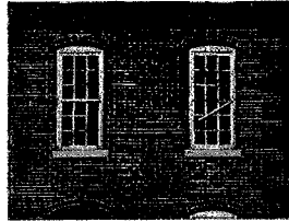
Historic Barn Deterioration
