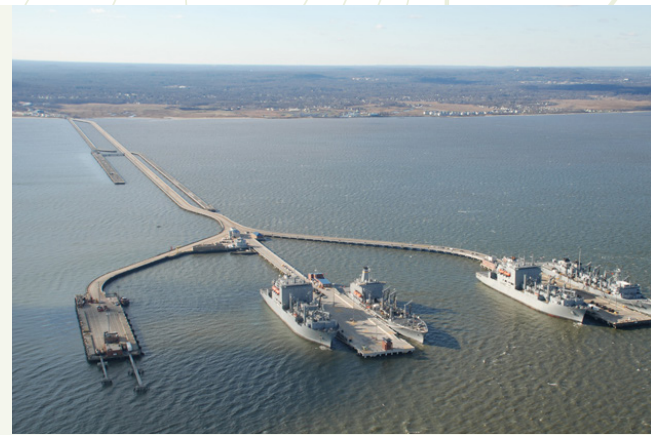
This 2.9-mile-long ammunition loading Pier Complex at Naval Weapons Station Earle is capable of berthing four 800-foot ships simultaneously.
