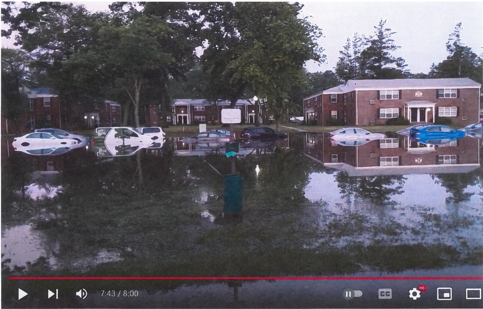
Flash Flooding at Eatoncrest Apartments - Eatontown, NJ - July 2021
